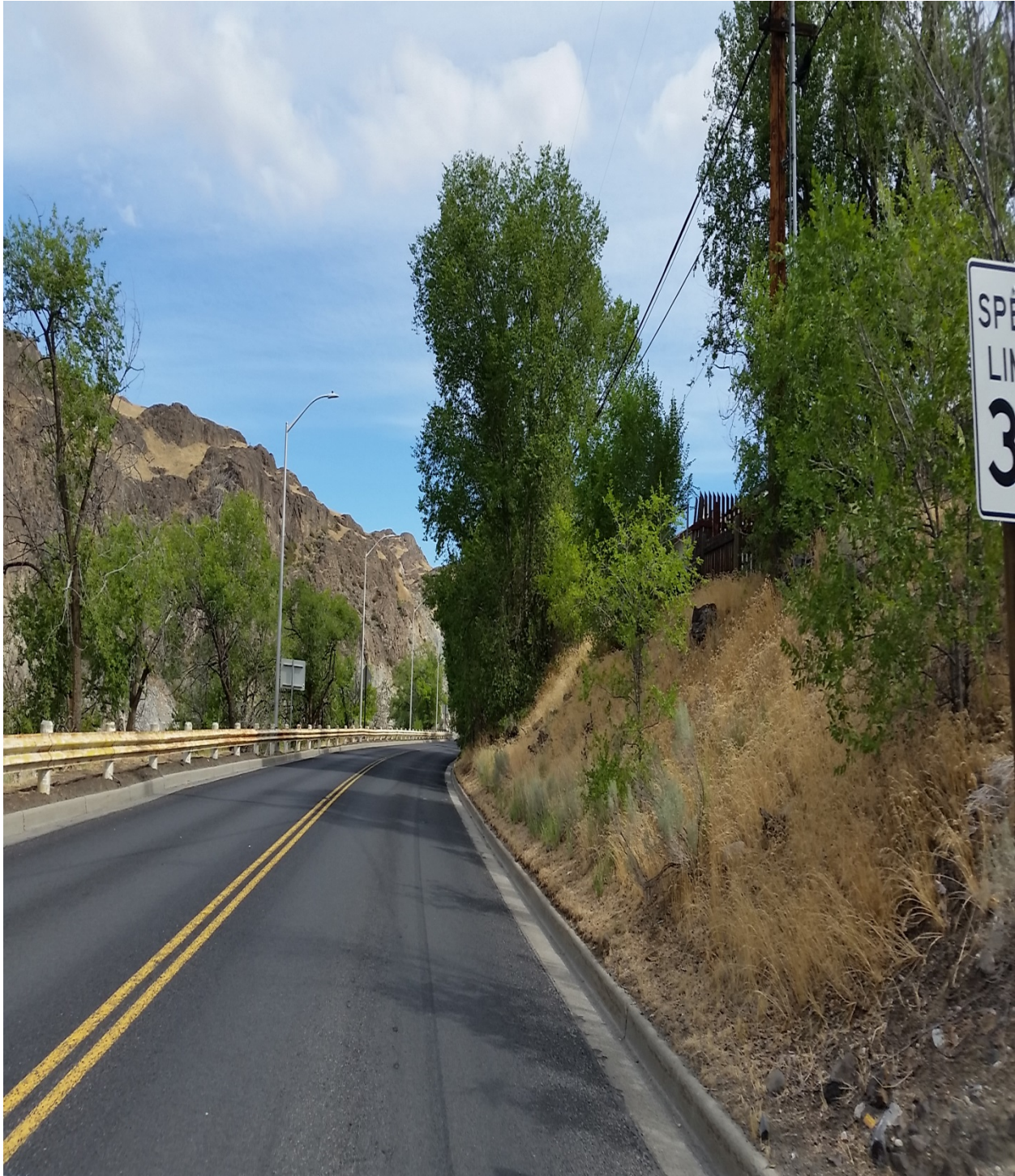
Photo 3: SR 155 Starting on Colville Indian Reservation/No Sidewalks 2015
